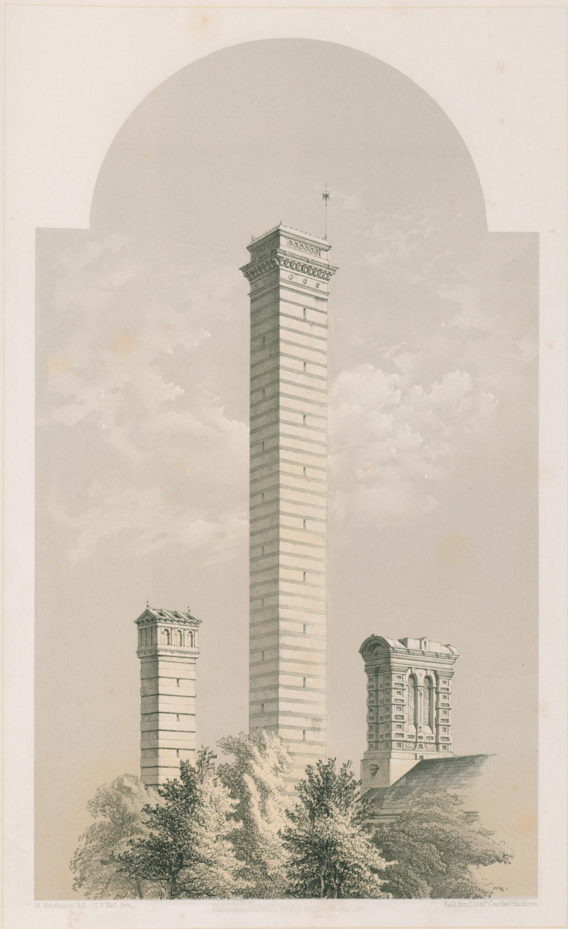
SHAFT FOR SEWER VENTILATION.
