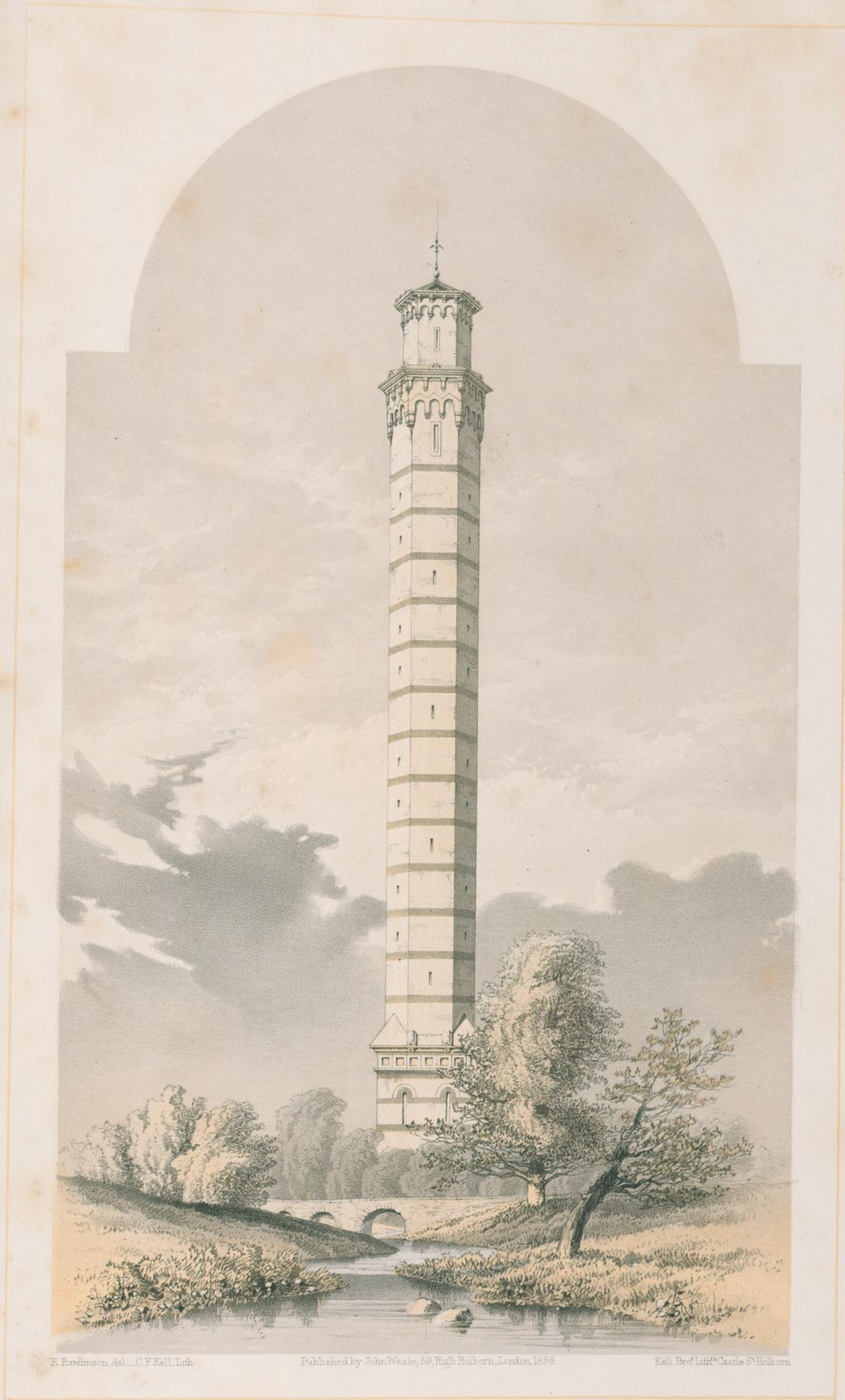
DETACHED CHIMNEY SHAFT .
