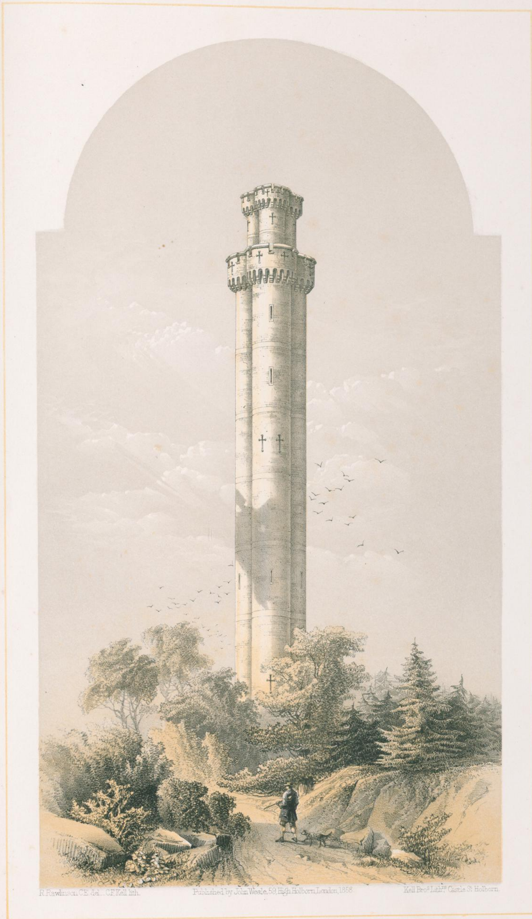
CASTELLATED CHIMNEY SHAFT.
