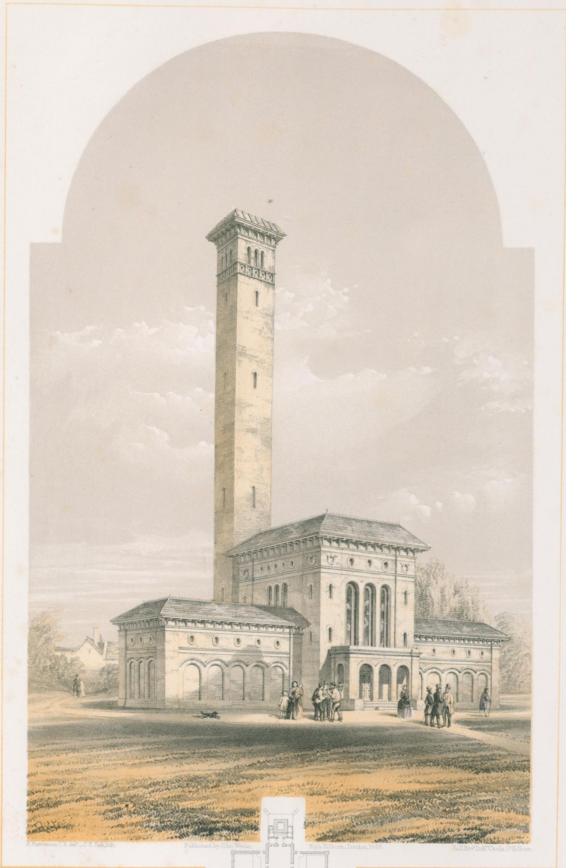
WATER WORKS. ENGINE HOUSE, BOILER HOUSES AND CHIMNEY SHAFT.
