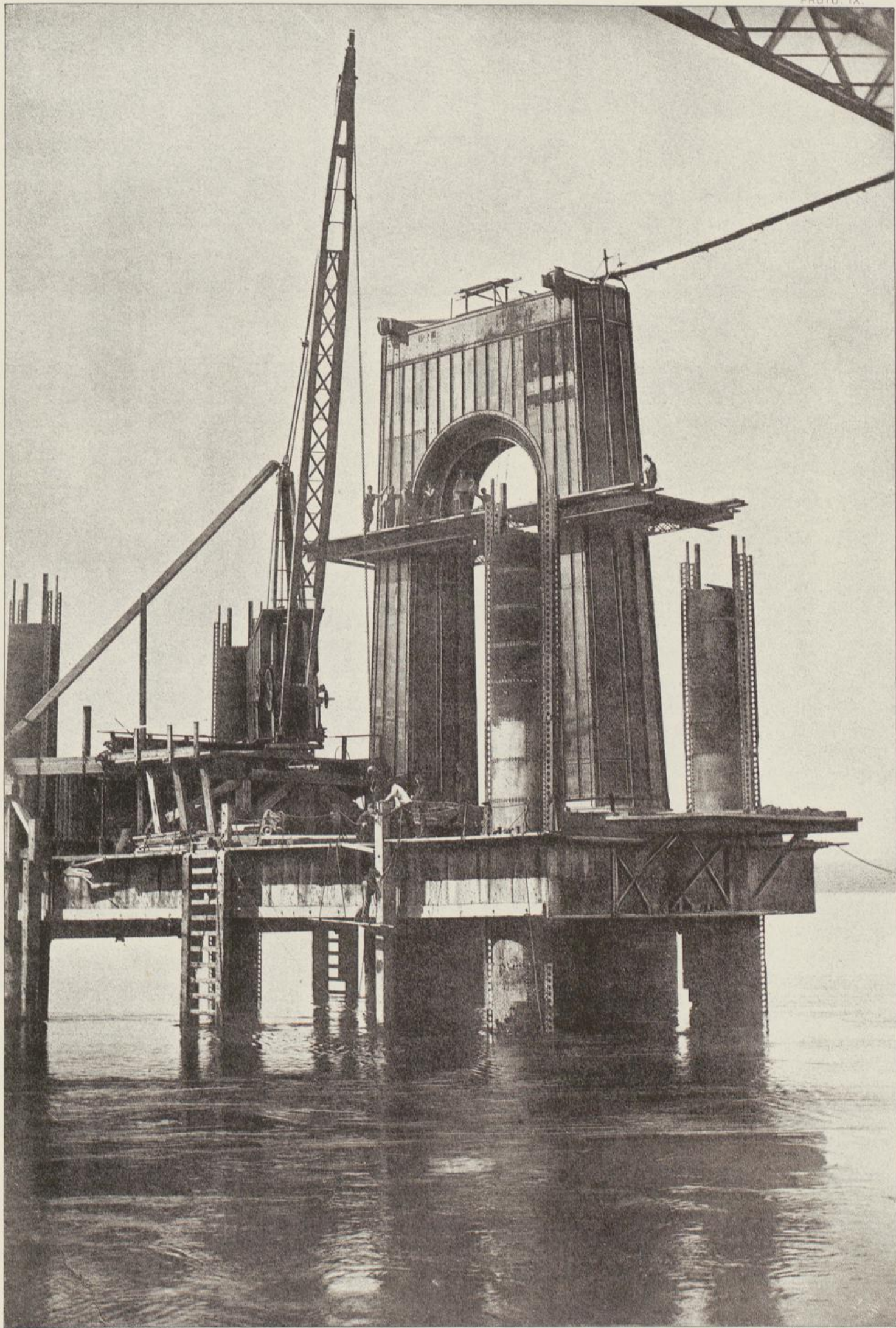
ERECTING THE SUPERSTRUCTURES OF PIERS - SOUTH SPANS.
